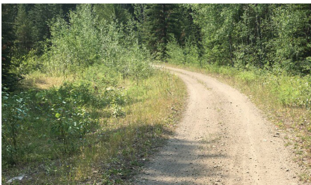
▼ Figure 36: Example of minor cupping/rutting of the trail tread within the track with of most OHVs
