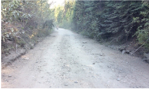
▼ Figure 34: Examples of poorly drained cut areas between Chute Lake and Myra Canyon Provincial Park
