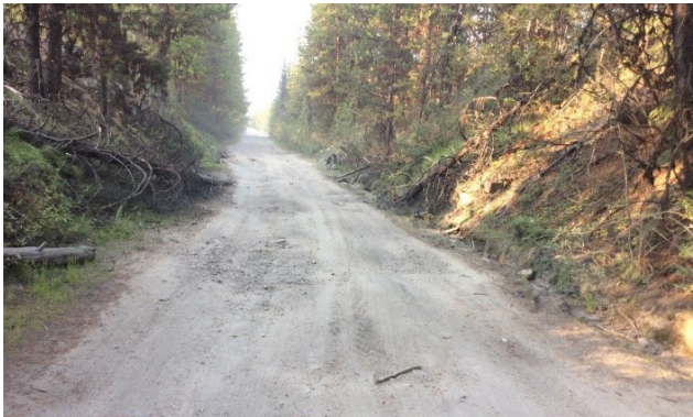
▼ Figure 35: Example of cupped trail where built up materials on the downslope side of the trail is preventing cross-flow drainage
