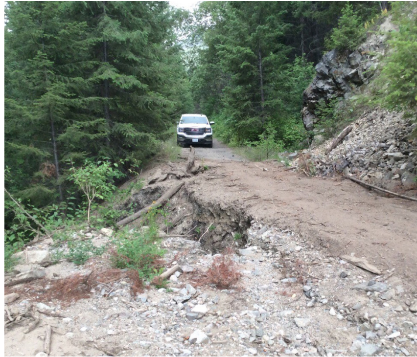
▲ Figure 38: Slope failure area caused by erosion and washout near Wilkinson Creek crossing
