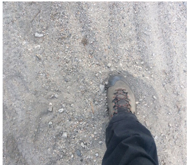
▼ Figure 33: Example of minor loose tread area north of Chute Lake
