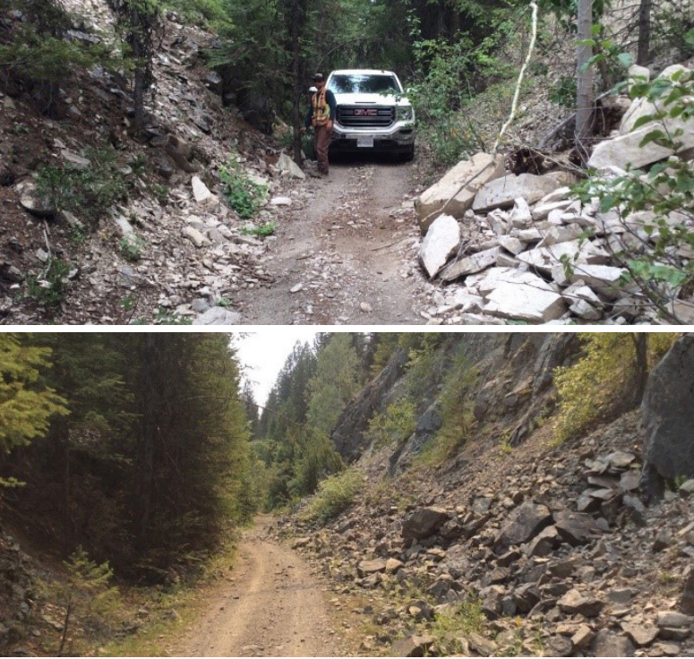
▼ Figure 37: Examples of rock fall onto trail tread near Arlington Lakes area
