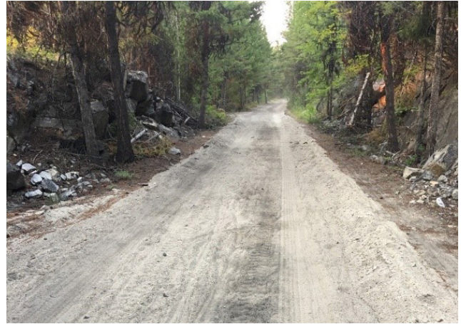
▼ Figure 32: Deep loose sand conditions approximately 2.2 km to 5.8 km south of Chute Lake
