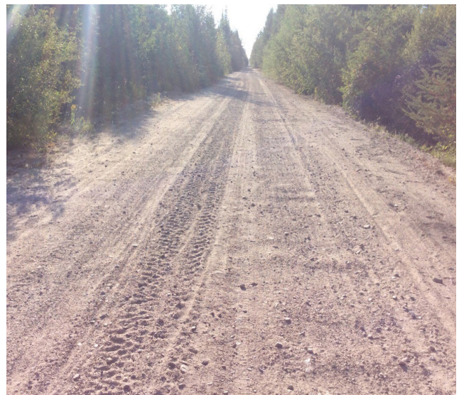
▼ Figure 33: Example of minor loose tread area north of Chute Lake
